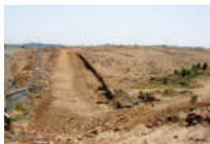
Construction of intra-back dam: excavation and casting
